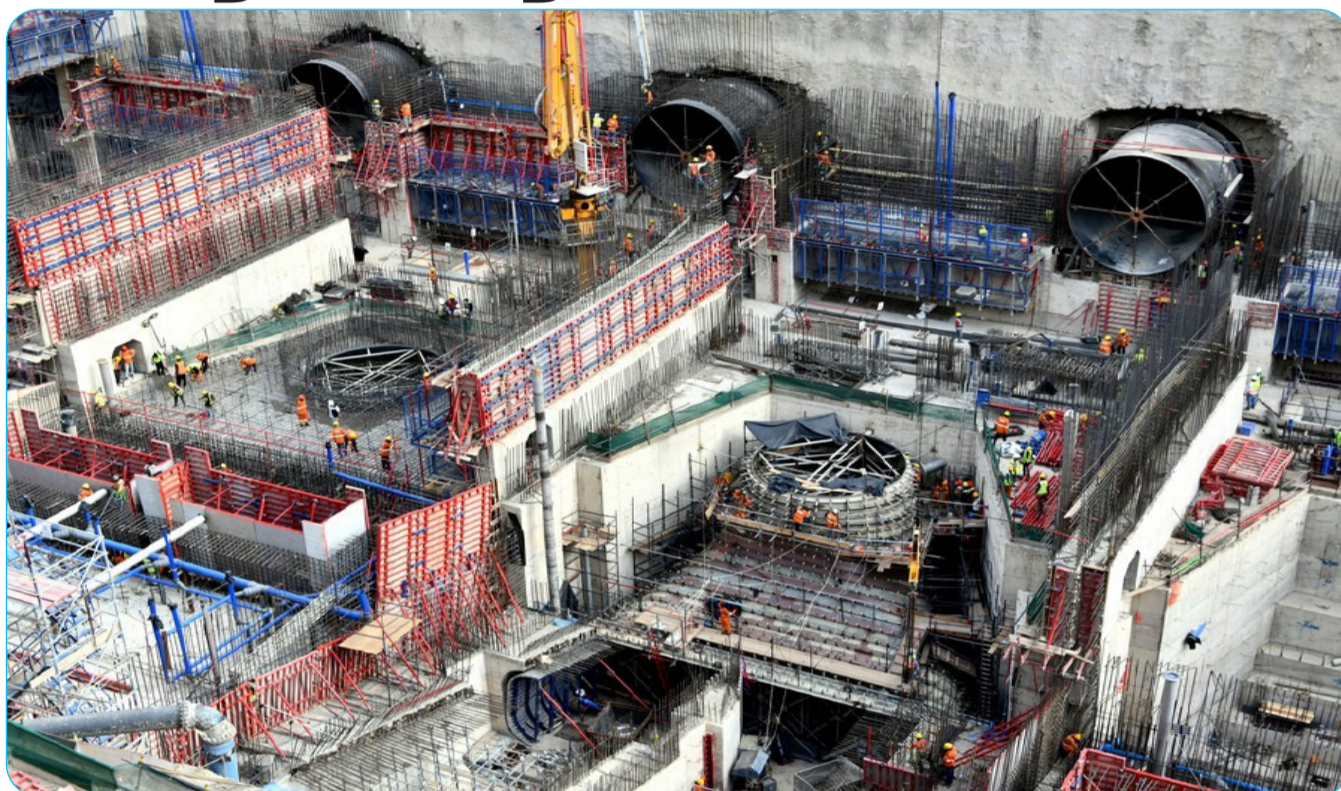
Construction of the Julius Nyerere Hydropower Plant Project. Photo: https://www.arabcont.com/English/project-596
